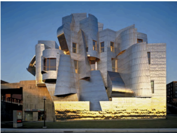
Frank Gehry Frederick R. Weisman Art and Teaching Museum, view of the west elevation, 1990-93, 2009-11, Minneapolis, Minnesota ©2015 Gehry Partners, LLP, photo ©2015 Don F. Wong
